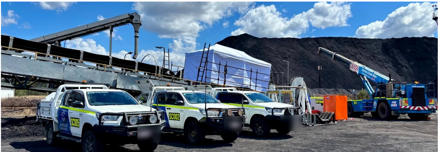
Superior site mobilisation and conveyor work.
