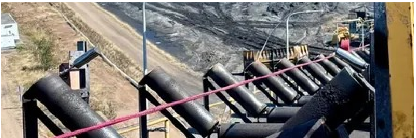
Belt and pulley installation on site. The photo does not identify the belt carcass.
