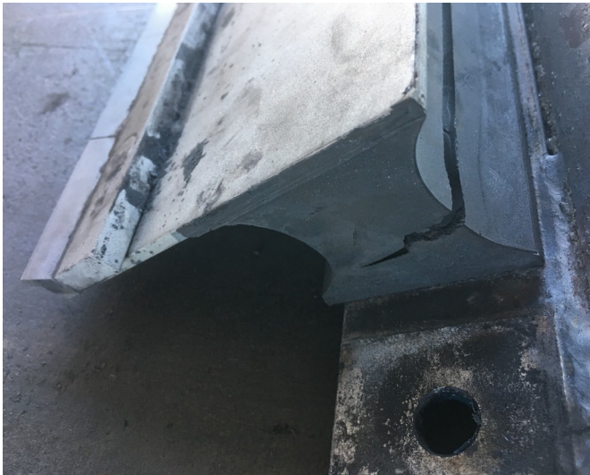
Cracked cleaner cushion requiring replacement and an attachment check.
