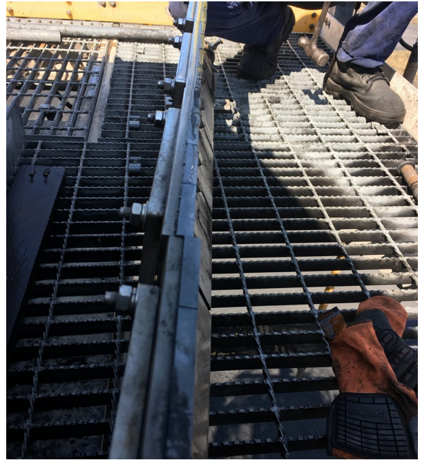
Cleaner components being serviced on site before refitting.
