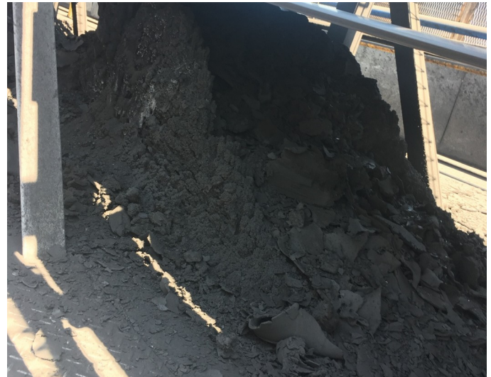
Accumulated material around the cleaning area restricts inspection and access.
